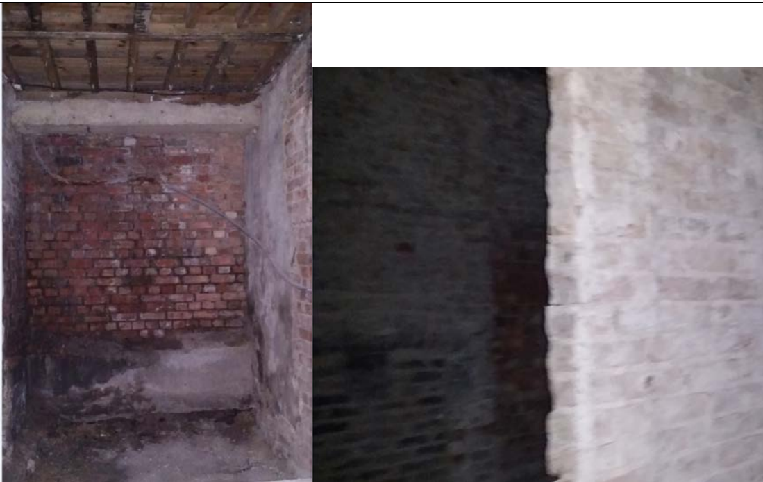
Basement of 32 Blomfield Villas (indicative of the size/state of all the basement spaces to be turned into 3 bedroom flats).
